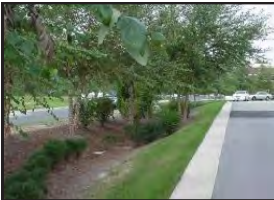
Flat curb edge with receiving vegetated swale.
