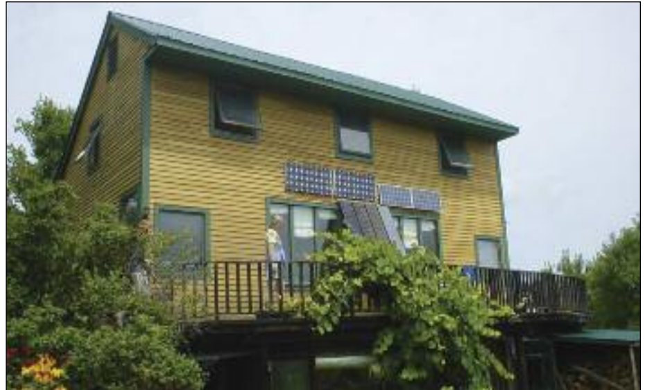
Building design is key. South-facing orientation provides much of this home's heat while the roof overhang, insulated curtains, careful placement of windows for x-ventilation and semi-earth-sheltered features keep it comfortable year-round.
