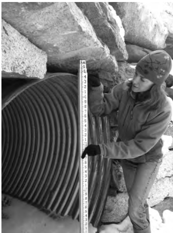
The author measures a culvert.
