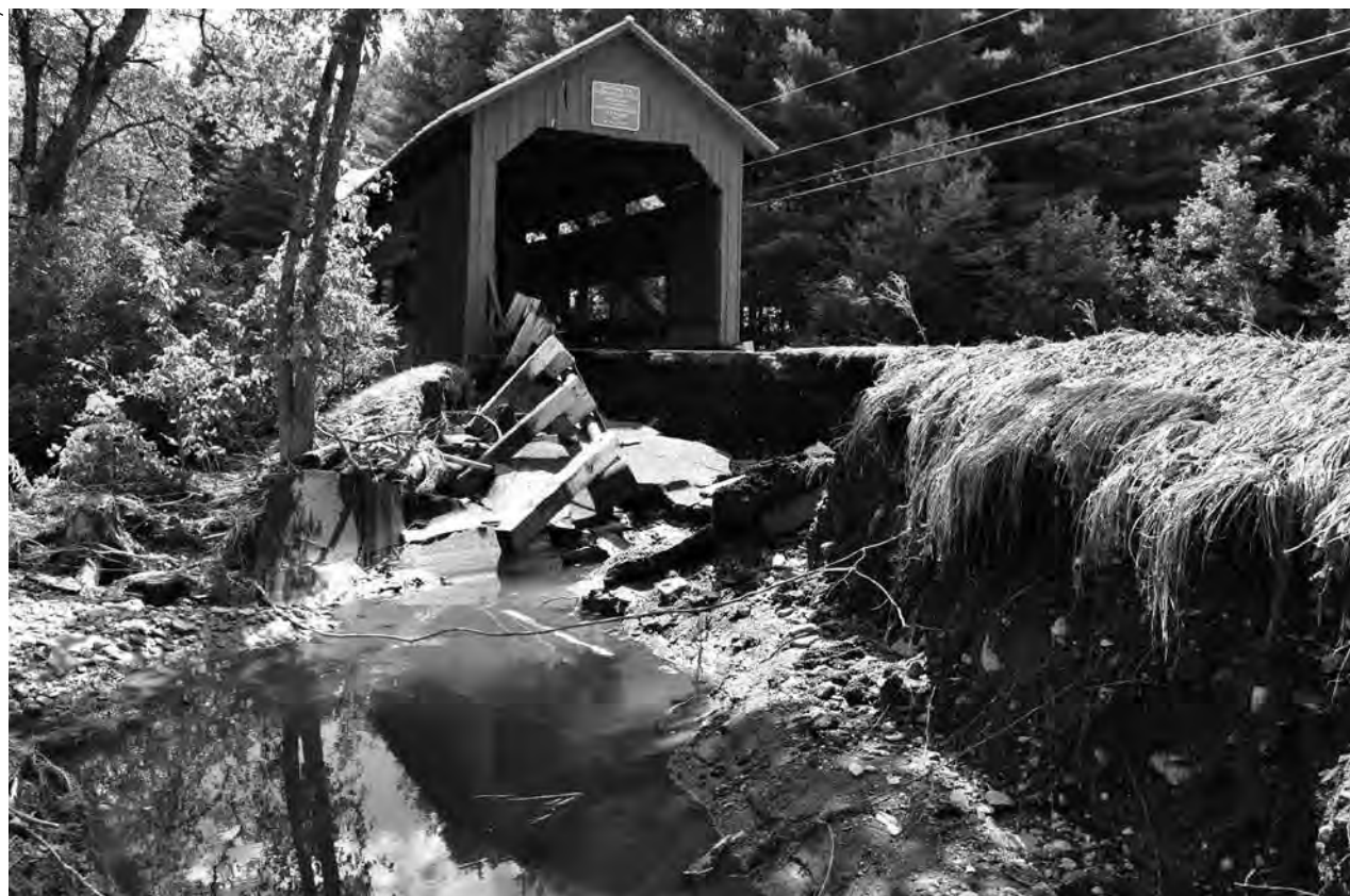
Erosion damage from flooding.
